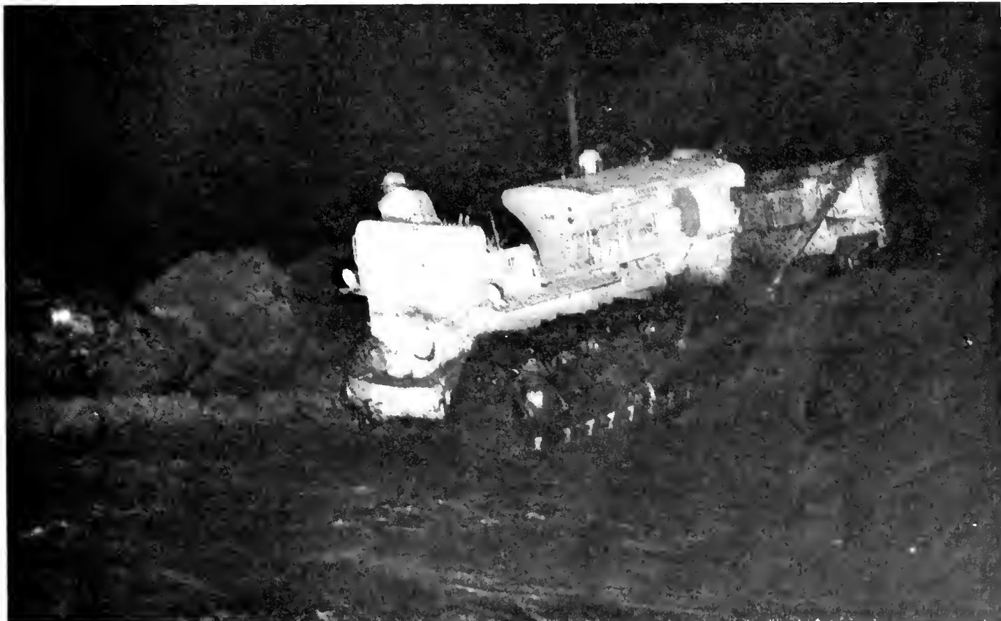
D8 dozer excavating for toe rock
